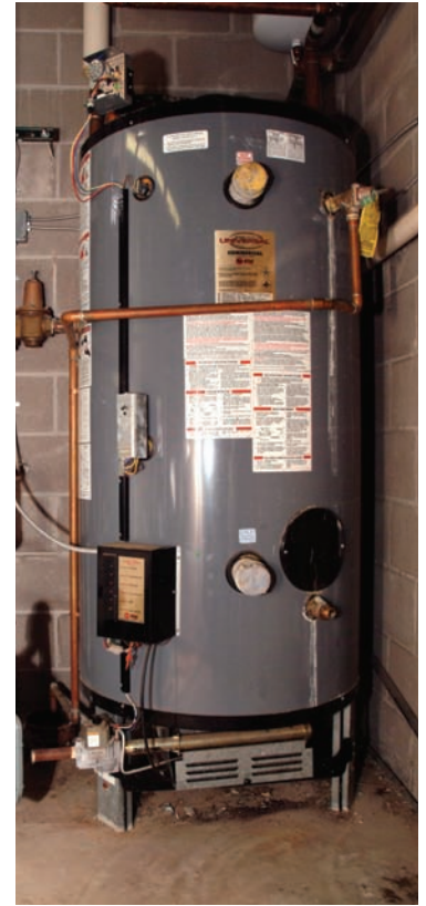
These 3 tankless natural gas water heating systems (above) replaced the 5-year-old 100 gallon natural gas water heater (right).
