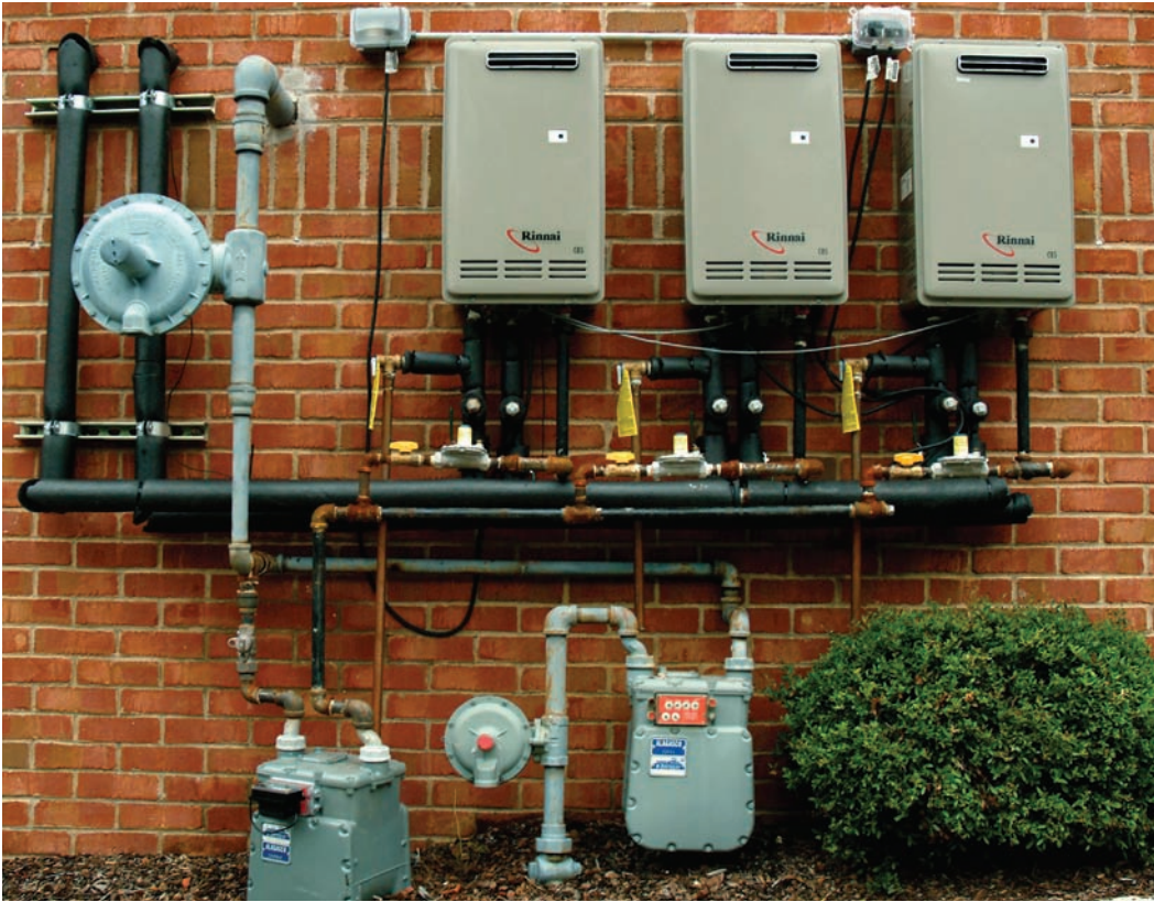
These 3 tankless natural gas water heating systems (above) replaced the 5-year-old 100 gallon natural gas water heater (right).
